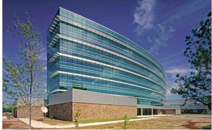
This building, owned by the Arkansas Department of Environmental Quality (ADEQ), benefits from natural daylight provided by ample glazing. However, when not carefully specified and designed, too much glass can lead to issues with heat loss or gain.
