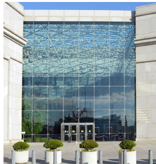
Federal Judiciary Building (Thurgood Marshall)
